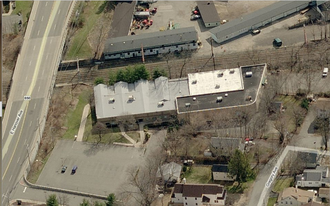
Aerial view of site
