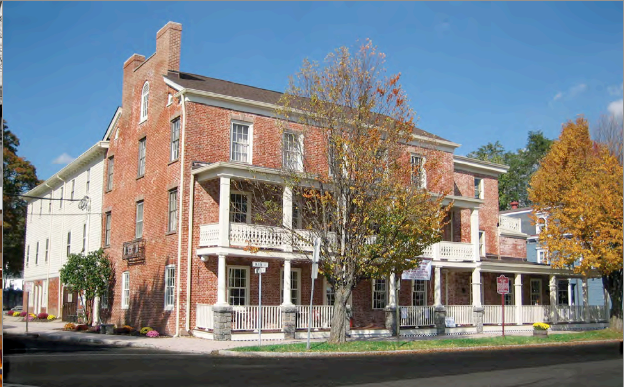
Phase One Completed Exterior
